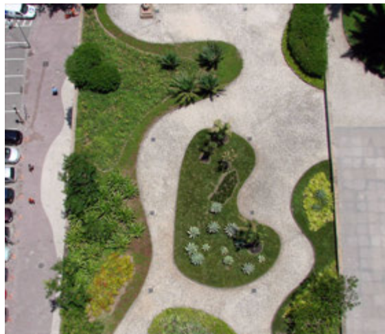
Bird's-eye view of an intensive green roof at the Ministries of Education building, Rio de Janeiro, Brazil.
