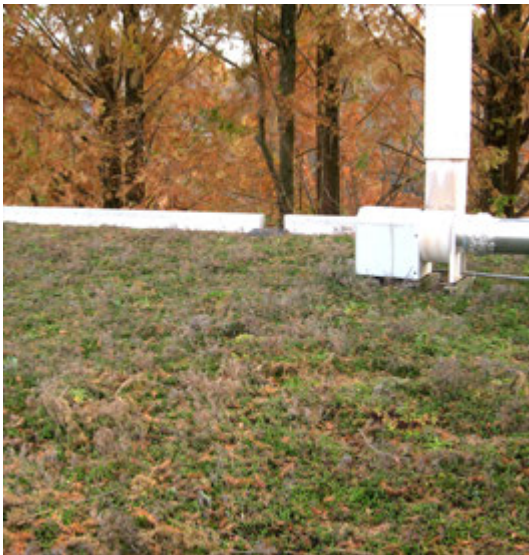
Autumn colors of an extensive green roof at the Sanford School, Hockessin, DE.
